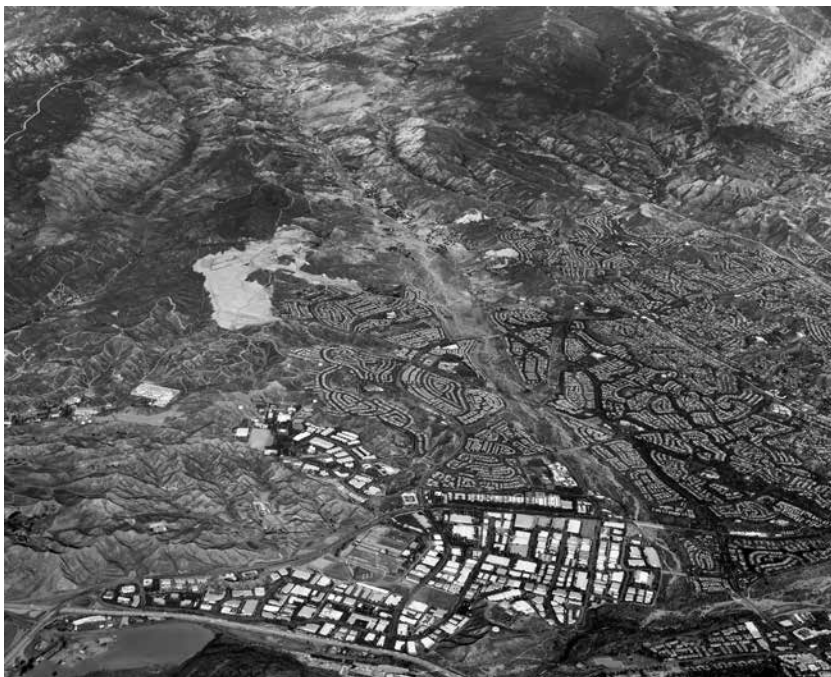
A view of most of the length of San Francisquito Creek, running southeast to the Valencia area of Santa Clarita. The Santa Clara River runs along the bottom of the picture, and the penstock of Power Plant #2 is visible toward the top. The St Francis Dam site is just above that.
