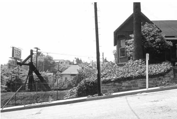
A house in Los Angeles across from Echo Park, seen here in 1977, had two oil wells in its yard. The pumps were run by cables running from a motor in the house.
