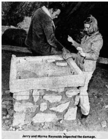
Jerry and Myrna Reynolds inspected the damage.
