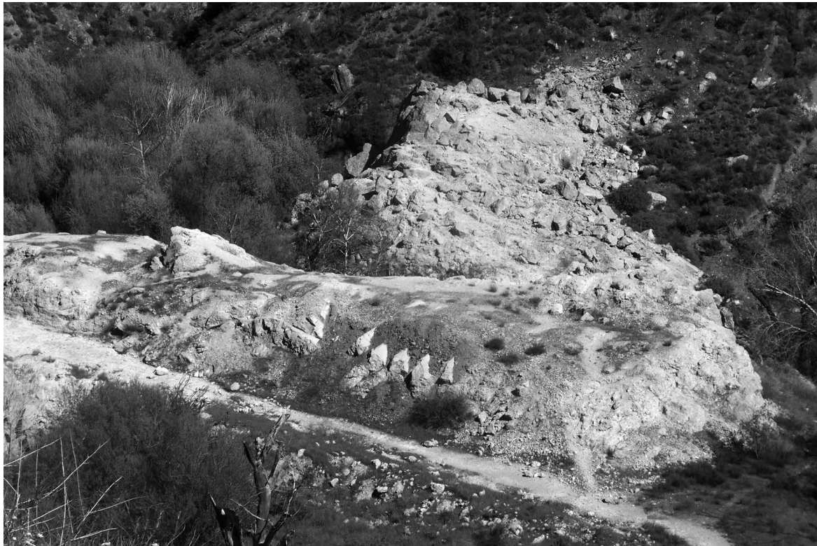
Remains of the St Francis Dam "Tombstone", showing evidence of the dam's staircase profile. For information on the upcoming tour, see page 4.
