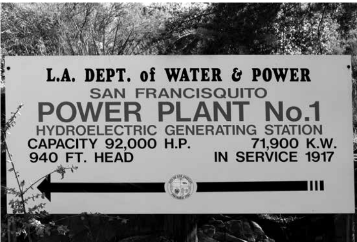
Entrance to L.A. Aqueduct Power Plant No. 1, located in San Francisquito Canyon above the dam site.
