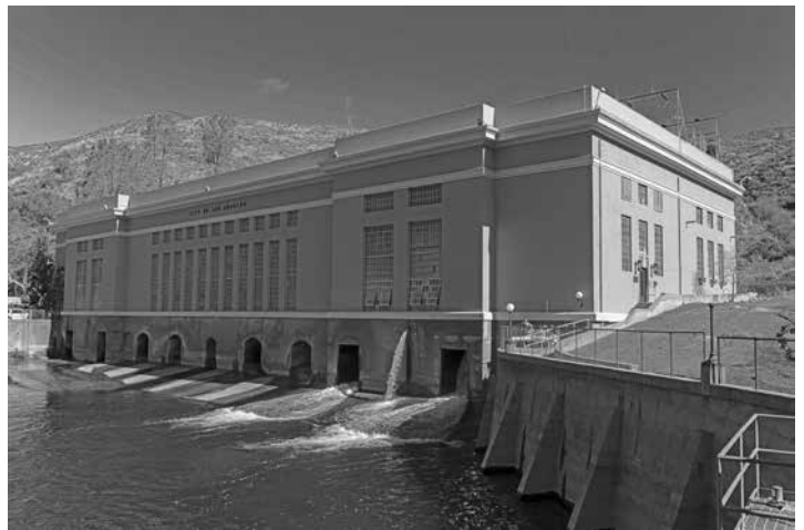
Power Plant No. 1. Inside is a chart on display showing the voltage transient when Power Plant No. 2 was destroyed.
