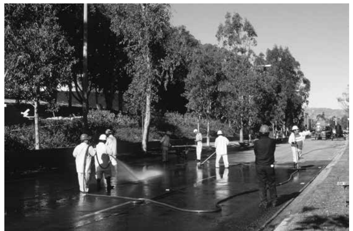
The 1994 earthquake ruptured an oil pipe under McBean Parkway
