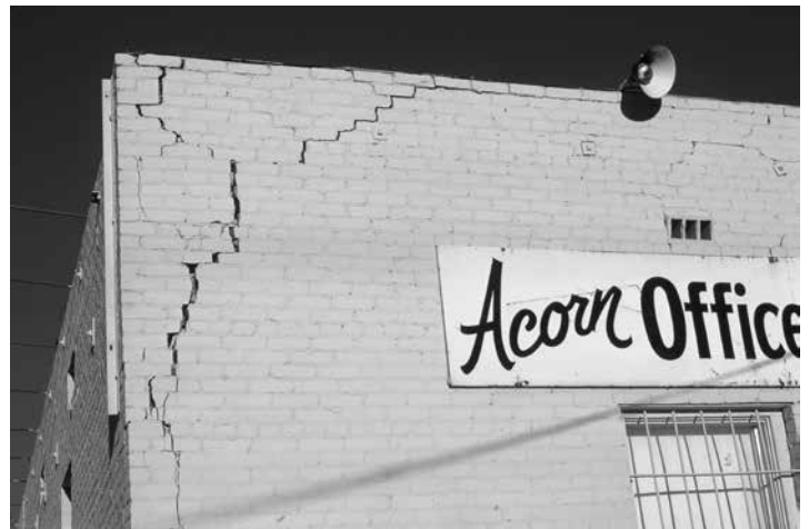
A building at San Fernando Road and Market St, 1971
