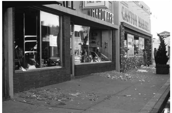
More recent earthquakes were messy, too. This is San Fernando Road in Newhall, 1971
