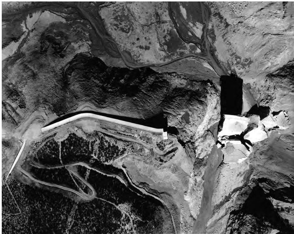
St Francis Dam after its collapse; see page 6
