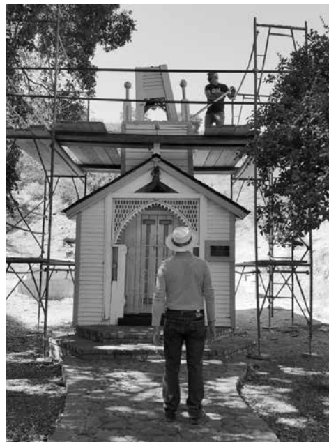
Due to structural damage, the steeple on the Ramona Chapel is being removed and replaced.
