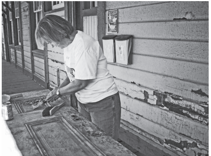
Linda Rehberger Preparing a Door at the Saugus Station for Refinishing
