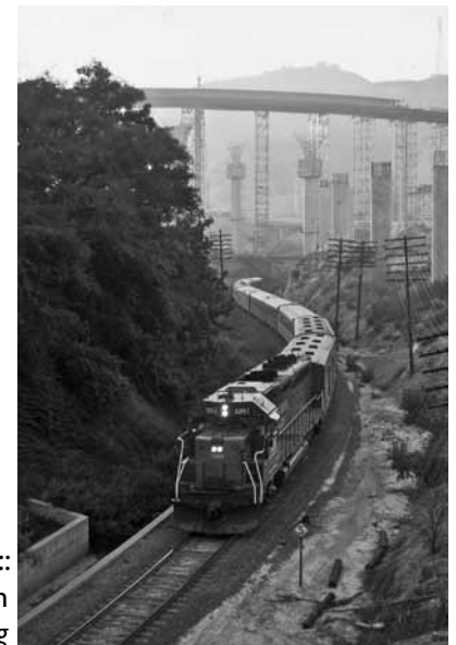
June 20, 1970: First Construction Photos by Gordon Glattenberg
