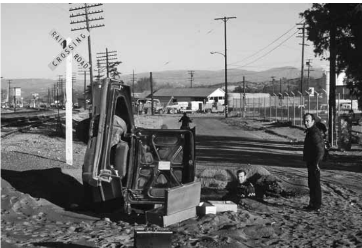
A sinkhole swallowed a car. This is just across the tracks from the present location of the Saugus Station
