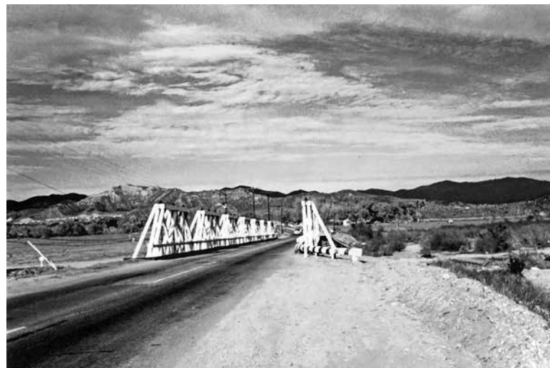
Bouquet Canyon Road bridge across the Santa Clara River, 1964. View looking north from where Chi Chi's is today. The only thing around was a Tapia Brothers fruit stand to the right of the photographer. The rest is all dirt where Best Buy, Lowe's, and Vons, etc are today.
