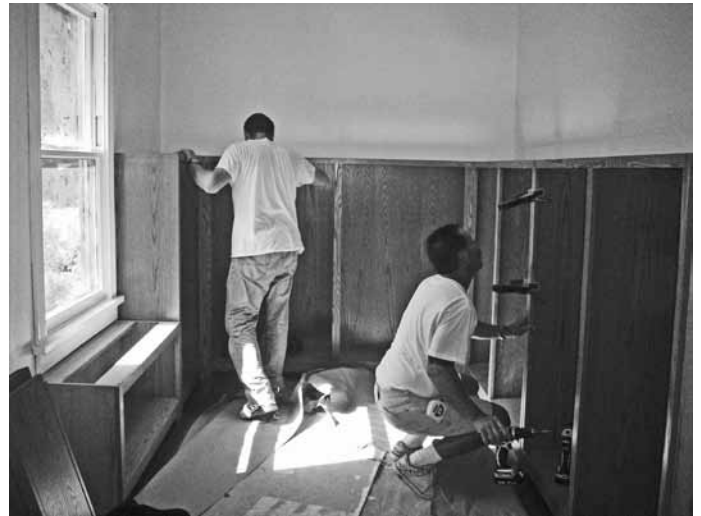
Installing Shelves in the Library
